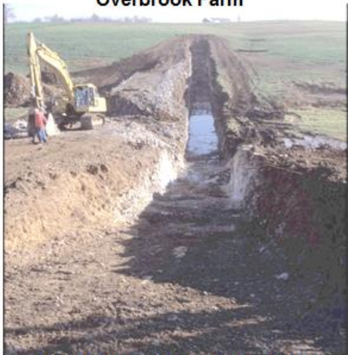
Cutoff trench to fresh bedrock
